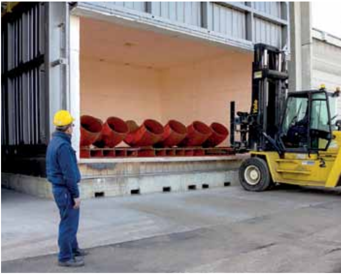
Two large furnaces outside and inside the plant
